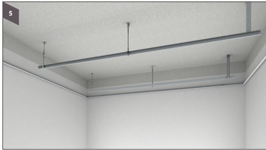
Fix the primary channel at 1200 mm spacing
