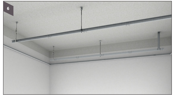
Hang the wire connecting clip WCC to the primary channel
