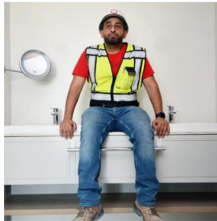
Man sitting on a cabinet fixed to USG ME drywall system. Check with USG ME technical team for the system design and allowable structural loads.
