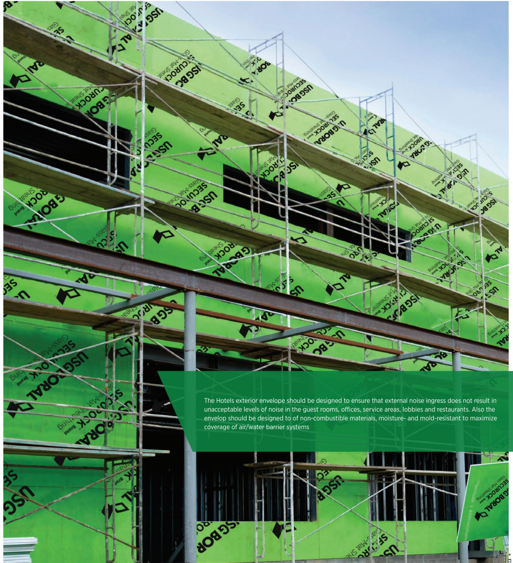
The Hotels exterior envelope should be designed to ensure that external noise ingress does not result in unacceptable levels of noise in the guest rooms, offices, service areas, lobbies and restaurants. Also the envelop should be designed to of non-combustible materials, moisture- and mold-resistant to maximize coverage of air/water barrier systems
